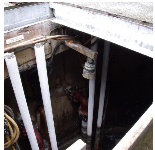
A typical wet well application.
